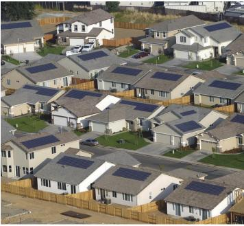
Often referred to by casual observers as solar panels, photovoltaic systems are single cells combined and connected to form PV modules. PV modules are manufactured with varving electrical outputs ranging from a few watts to more than 100 watts of direct current. The modules are then connected into PV arrays to power electrical devices.
